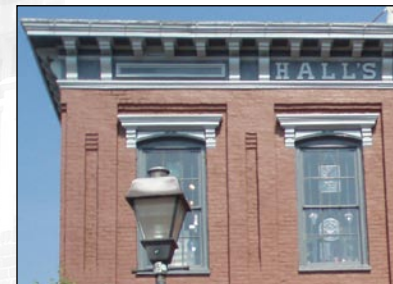
Built-up cornice on brick masonry
