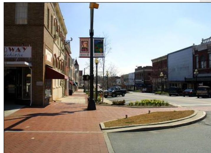
Brick pavers crosswalks with concrete edging
