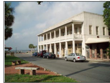
Masonry hotel with continuous balcony
