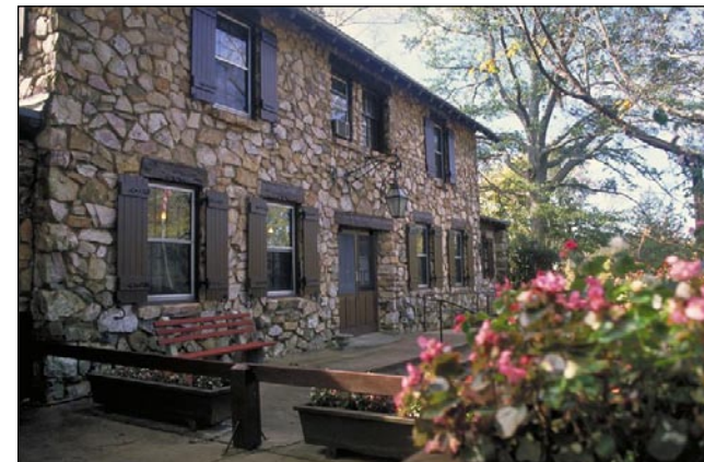
Stone building at Roosevelt StatePark
