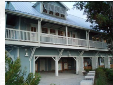
Wood building with continuous porch
