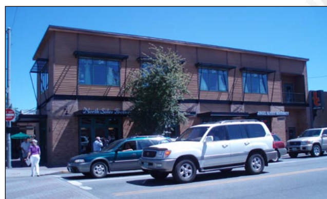
Wood and masonry building
