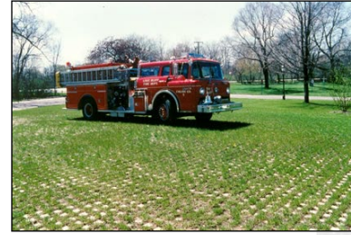
Pervious parking with "Grasscrete"
