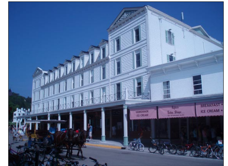
Long building with pattern created by dormers
