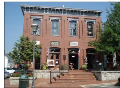
Victorian Two-Part Commercial Block - Hall's Block, 1883
