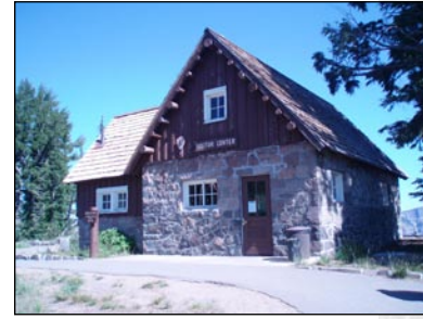
Masonry and wood building
