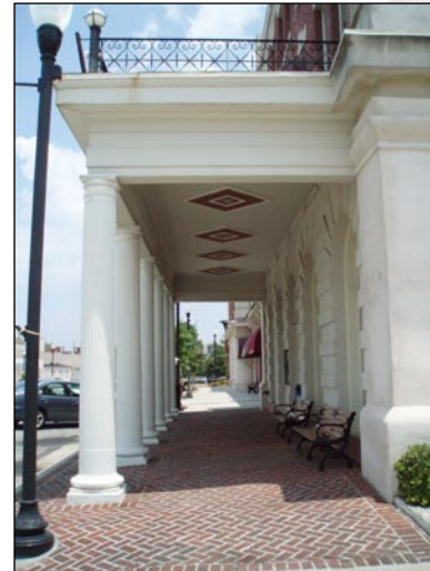
Porch covering the sidewalk
