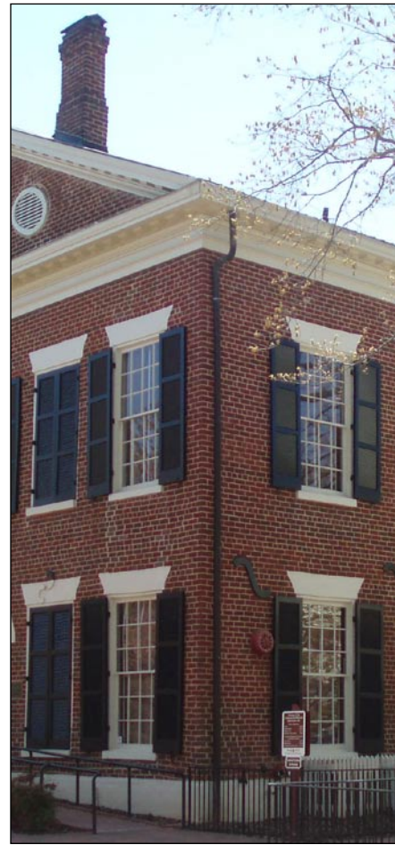
Stone lintels and sills, operable shutters
