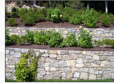
Stone retaining wall
