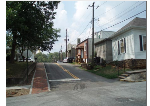
Brick sidewalk on one side
