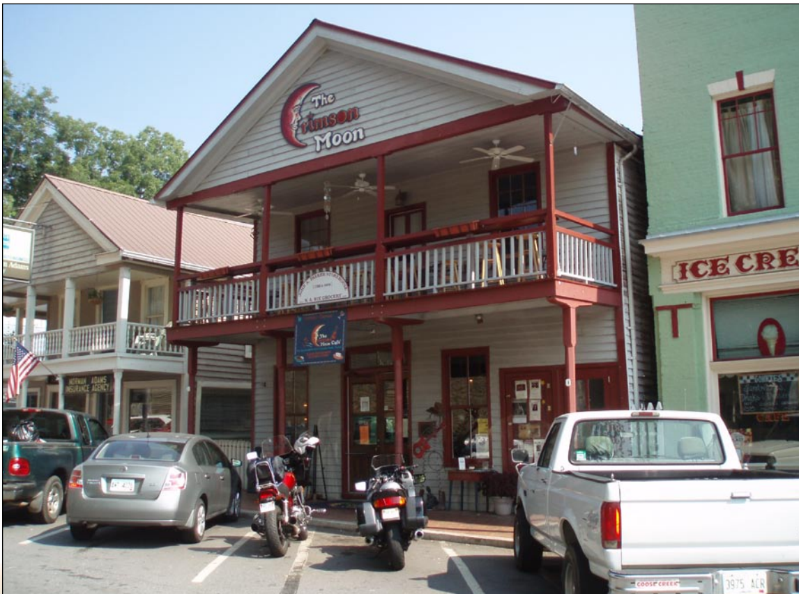
Figure 2.15: Public Square Architecture
