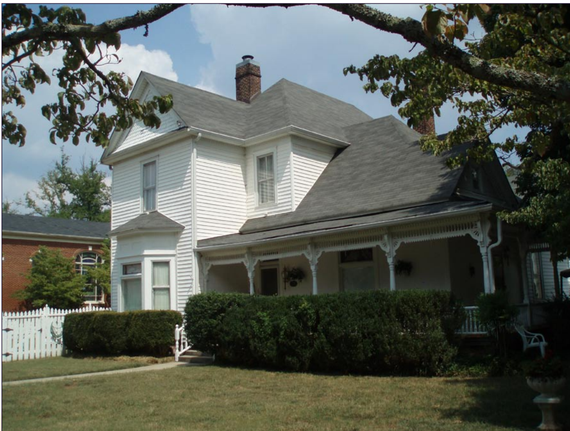
Figure 3.12: Park Street House
