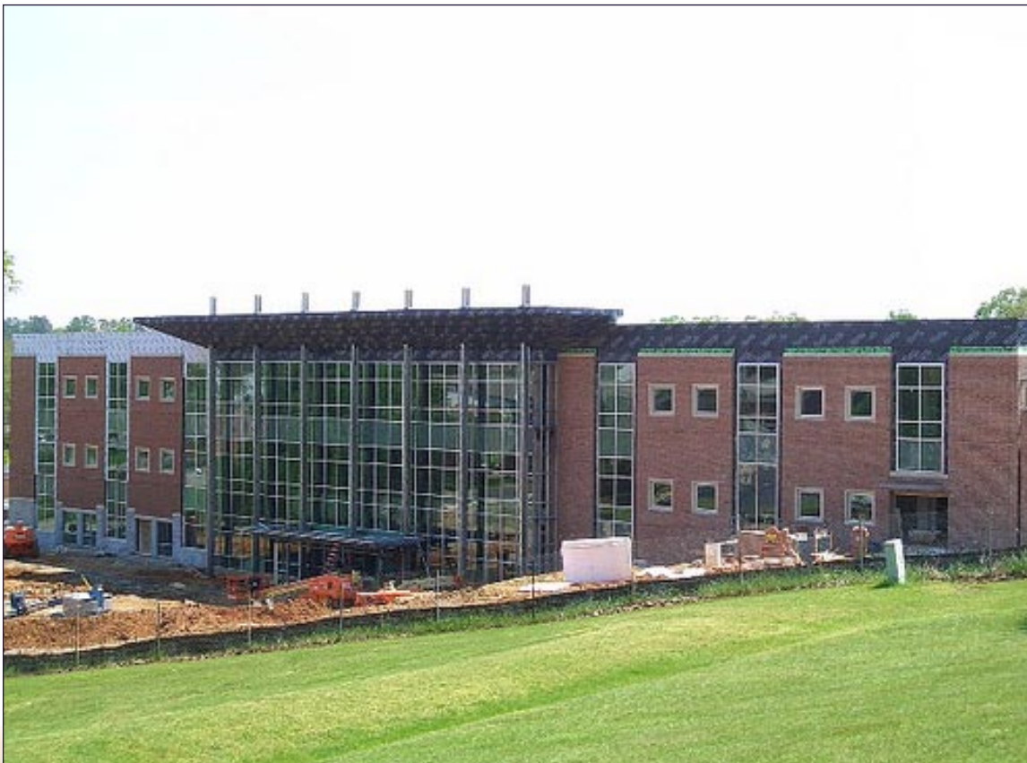
Figure 3.49: New Campus Library Construction Photo
